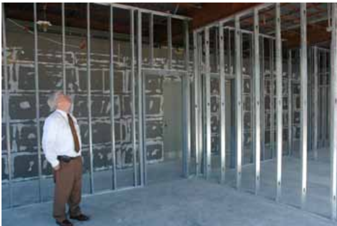
Executive Director Perry Roquemore surveys the office expansion project at League headquarters (November 6, 2010).
